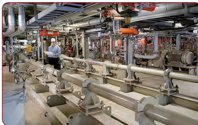
Multistage centrifugal pumps are cost-effective solutions in high-pressure fluid handling applications
